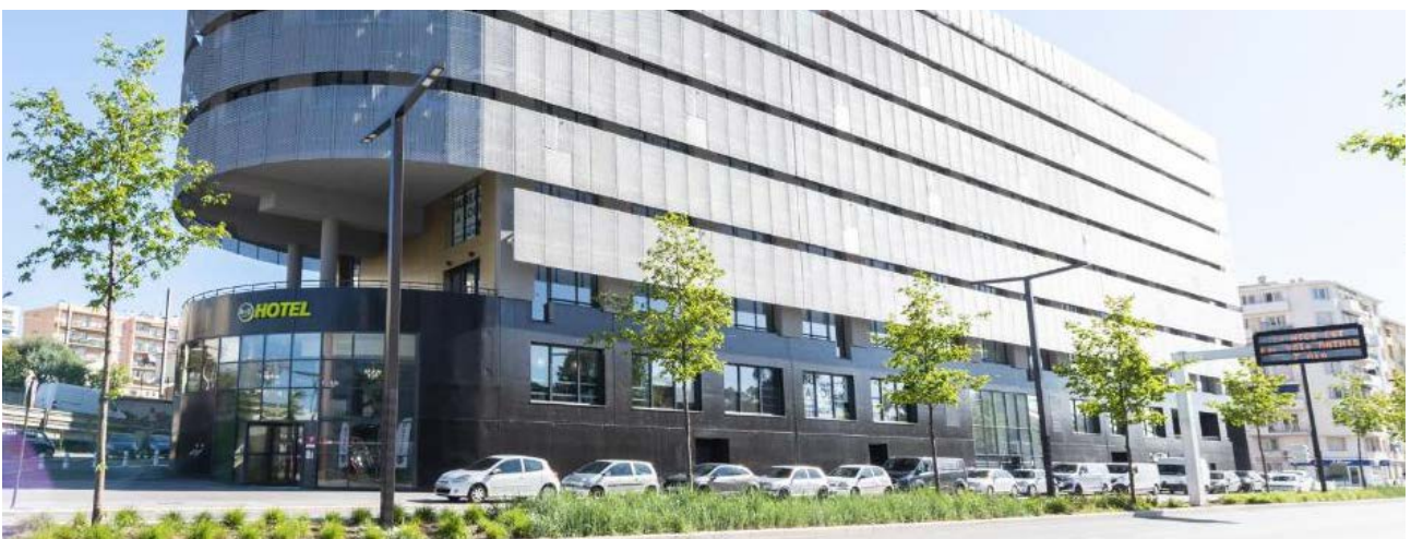
Hotel B&B Nice Aeroport Arenas ©Primonial REIM France
