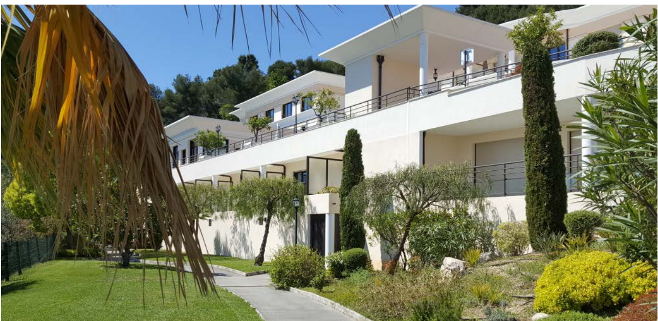
Beausoleil EHPAD Korian ©Primonial REIM France
