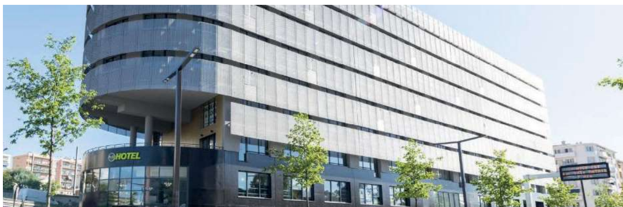
Hotel B&B Nice Aeroport Arenas ©Primonial REIM France
